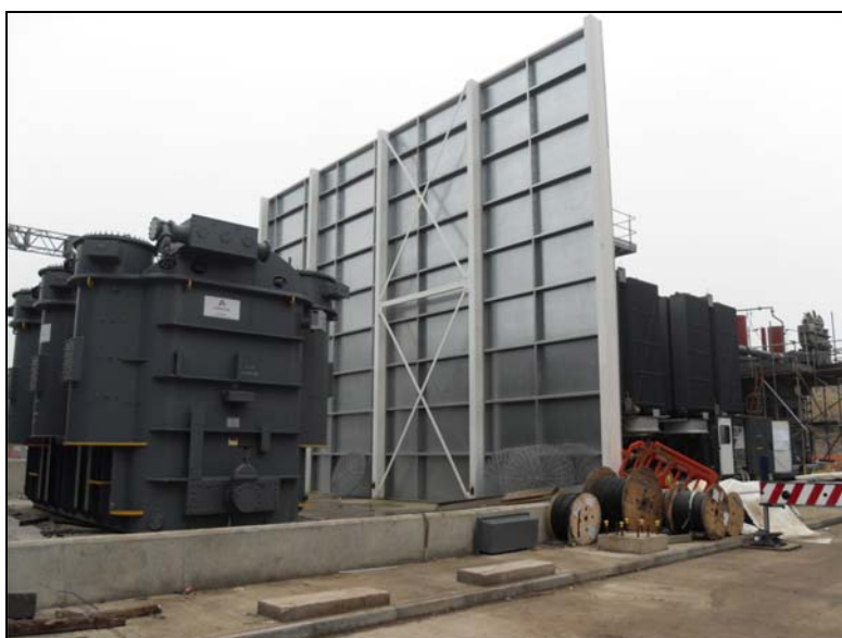
Promat DURASTEEL® barriers protect against transformer blasts
